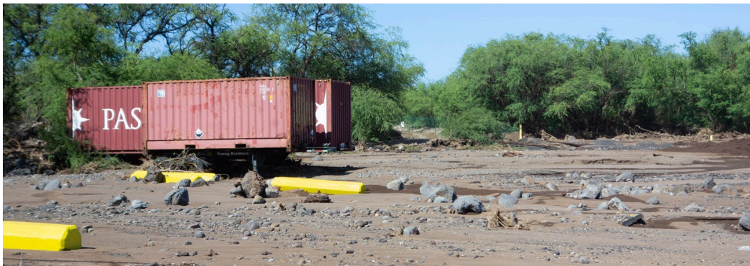
Large boulders deposited on container yard at south gate and adjacent to harbor office, 5/14/2024
