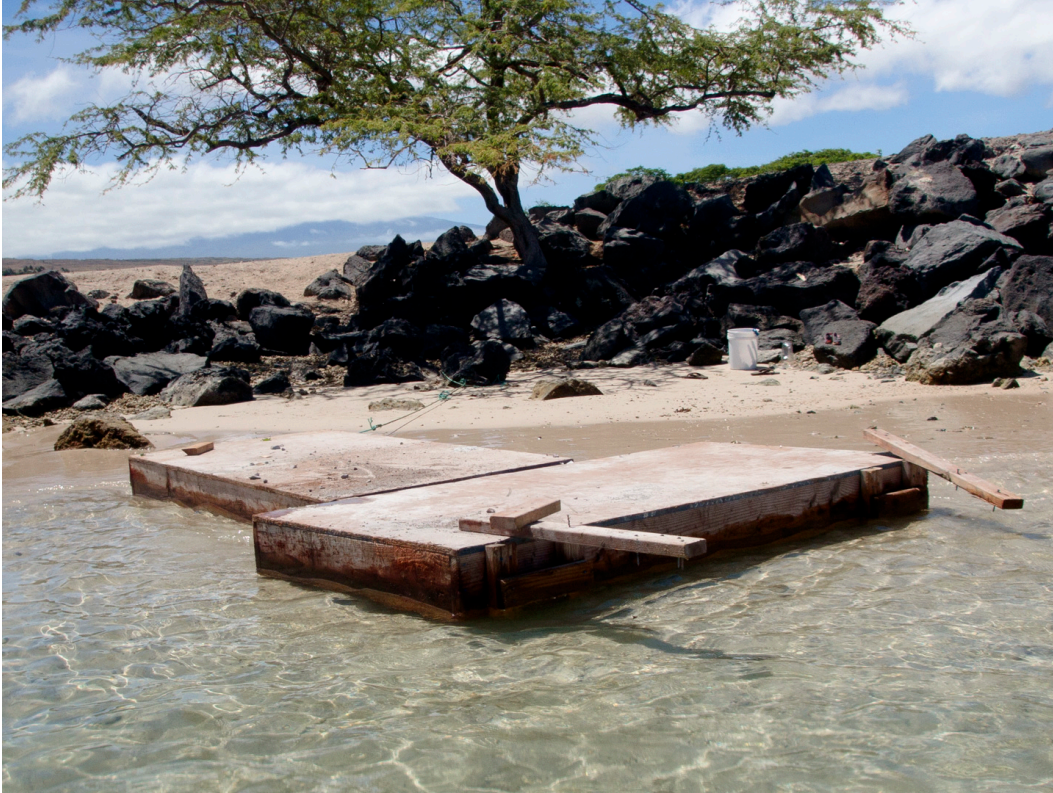
Two floating temporary construction platforms broke free and ended up on a small beach inside the harbor, 6/12/2025
